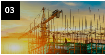
03 Managing construction risk & insurance programs with confidence
