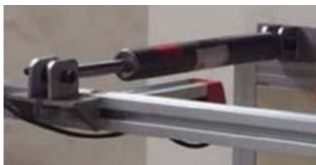
Fig. 5 Viscous fluid dampers provided on top of Stockers (Photos courtesy of Lockton client & NYCU)
